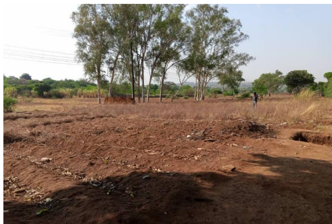
Figure 5: land preparation in progress, Chivamba Extension Planning Area, Lilongwe East
