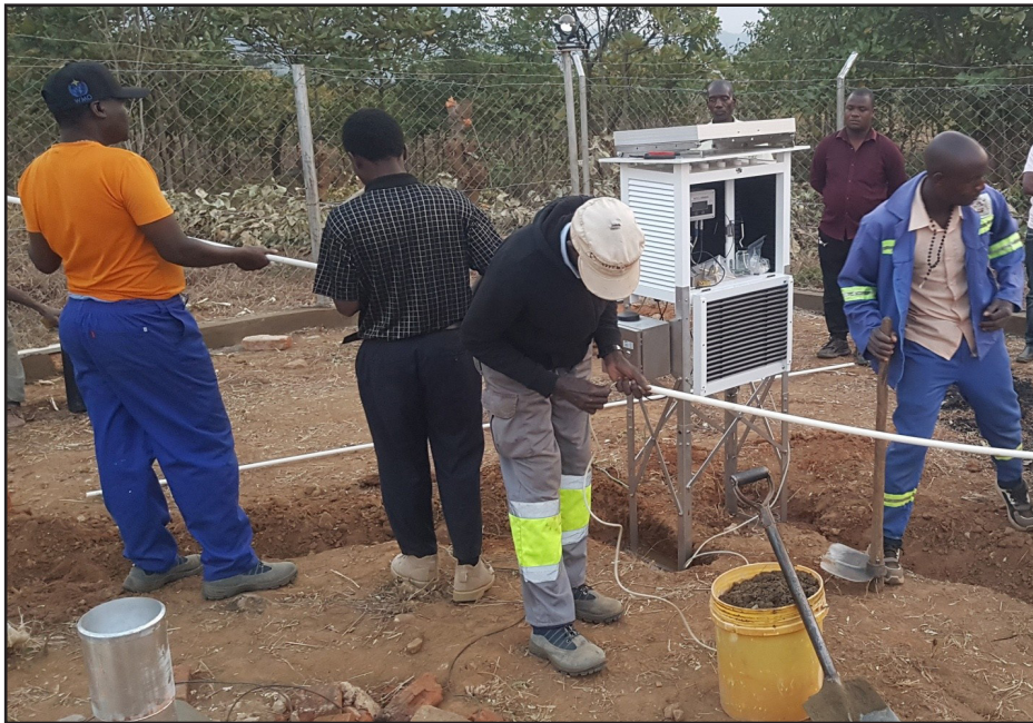
Installation work at the new Neno weather station at the old Neno airfield.
