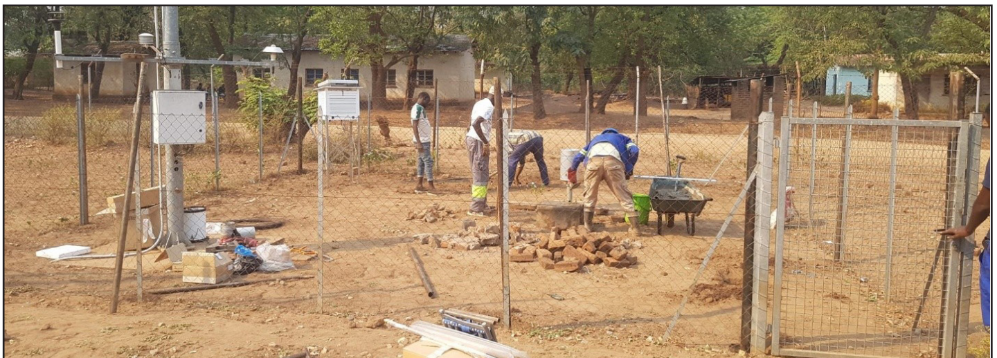
Work under way at the new Nsanje weather station at the district Agriculture
