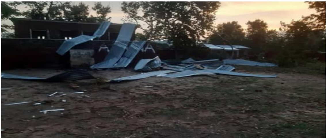
Figure 46: Destroyed Mpotola Primary School in Ntcheu district (Times360 19 November 2025)
