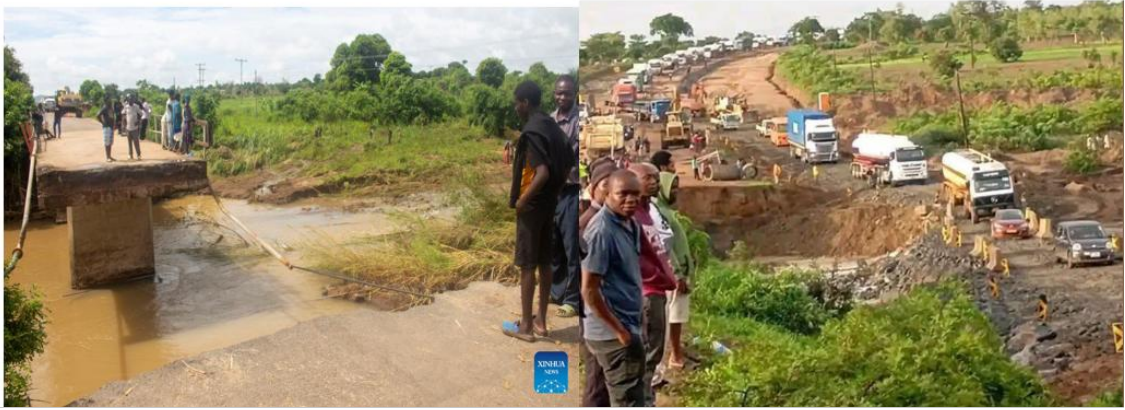
Figure 23: Damage due to floods in Nkhotakota December 2025.
