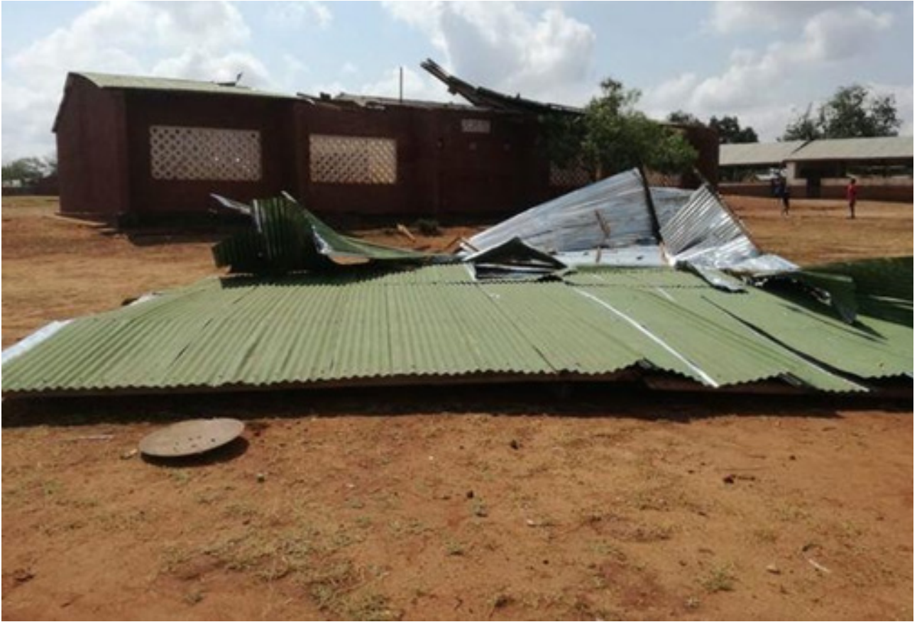
Figure 29: Primary school roof blown by strong wind in Mangochi, November, 2022
