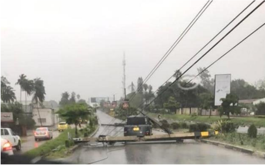
Figure 32: A toppled electric pole in Blantyre as a result of heavy rainfall during Tropical Cyclone Freddy
