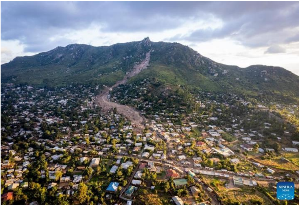
Figure 24: Residential area in Blantyre, Malawi (aerial view) after being struck by a mudslide during Tropical Cyclone Freddy. Photo by Joseph Mizere/Xinhua
